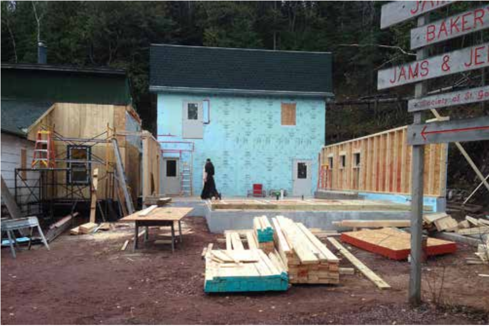
Expansion Phase I in progress.
