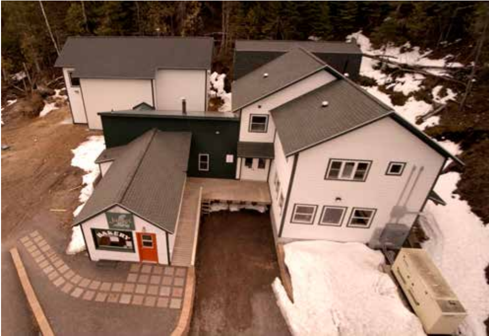
Phase II Complete
