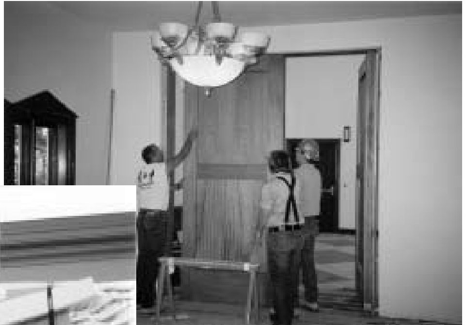
Workmen install the Great Doors between vestibule and church.
