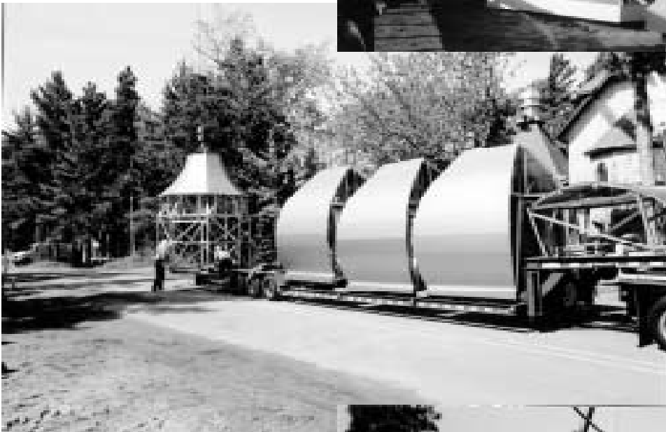
Sections of the main Dome arrive.
