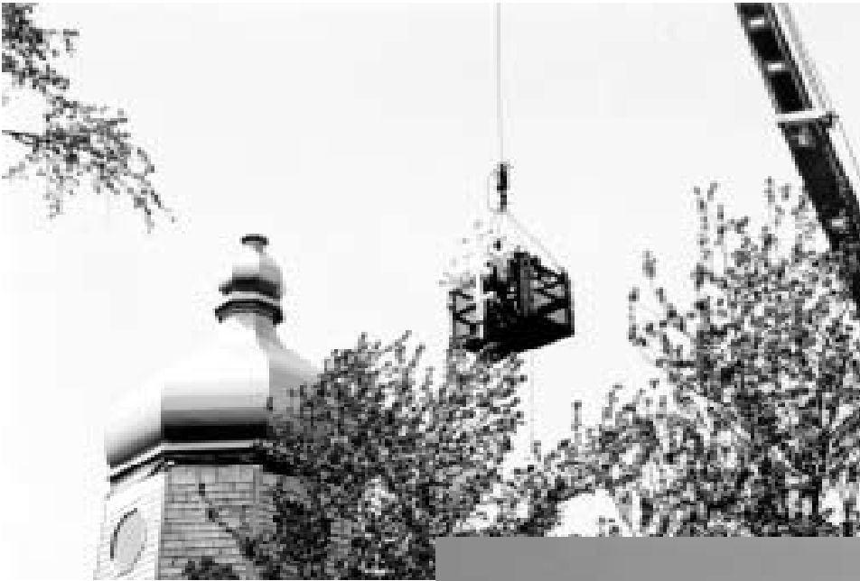
The Crane lifts workmen toward the main Dome for placement of the Cross.
