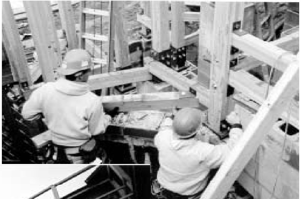
Workmen assemble the Belltower framing.
