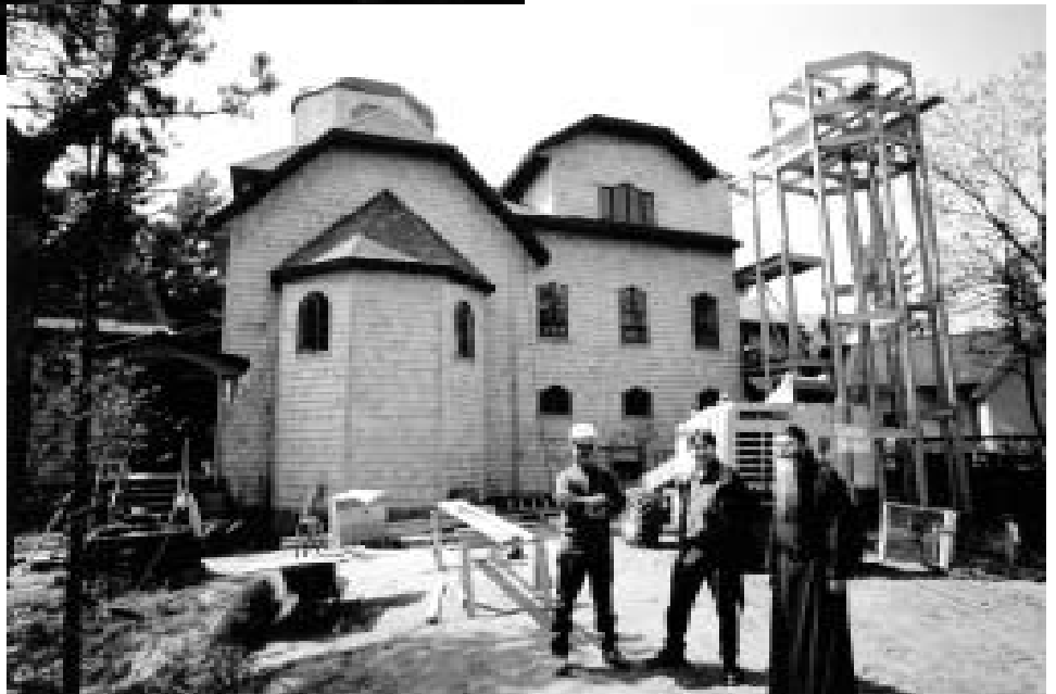
Architect, Page Onge, pays a visit to the building site.
