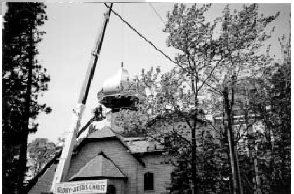
Assembled lower portion of the main Dome is raised into place.
