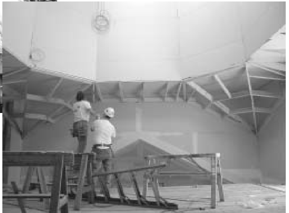
On scaffolding raised under the octagon, workers frame the tower vaulting.
