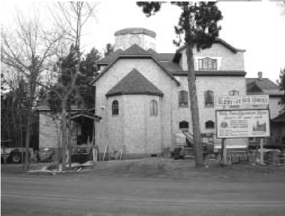
Nearly completed building awaits springtime erection of dome and bell tower.
