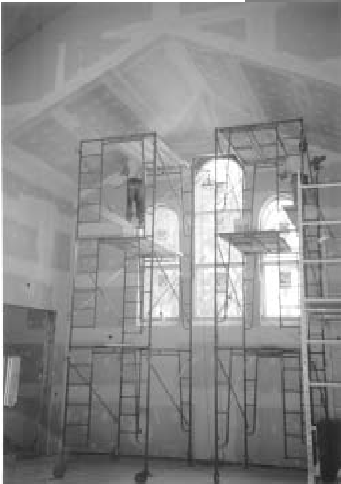
Workmen finish drywall at the West windows of the church.
