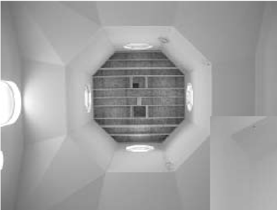
Octagon ceiling awaits final installation of the dome before completion.
