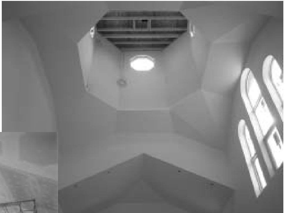
Looking East, into the Tower.
