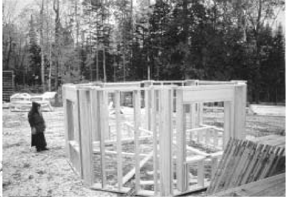
The Newly framed Tower Octagon in the Jampot parking lot, awaiting transportation to the building site.
