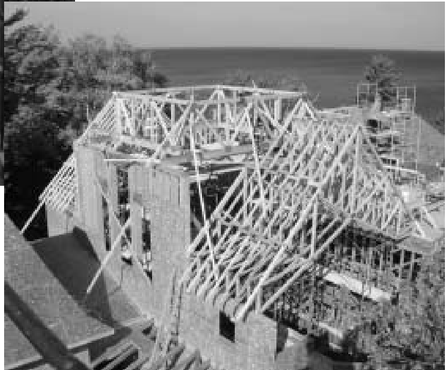
An eagle eye view of the Church roof and Tower trusses.
