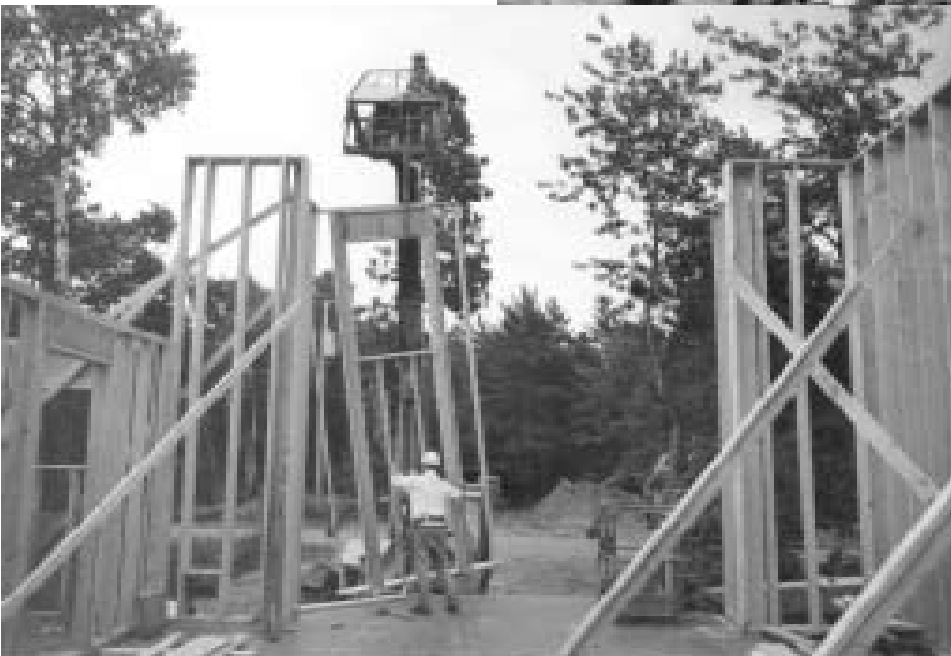
The Northeast wall of the Apse goes into place.
